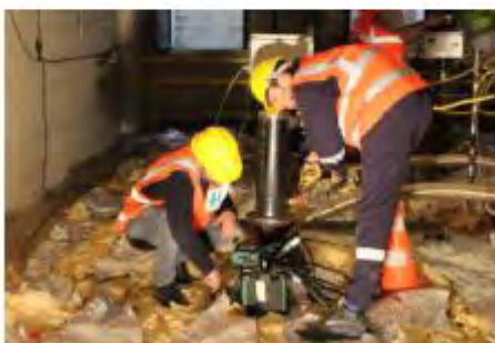
4. Installation of the Smart™ burners
